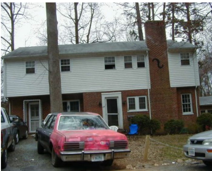
526 Valley Road (1935, altered)
