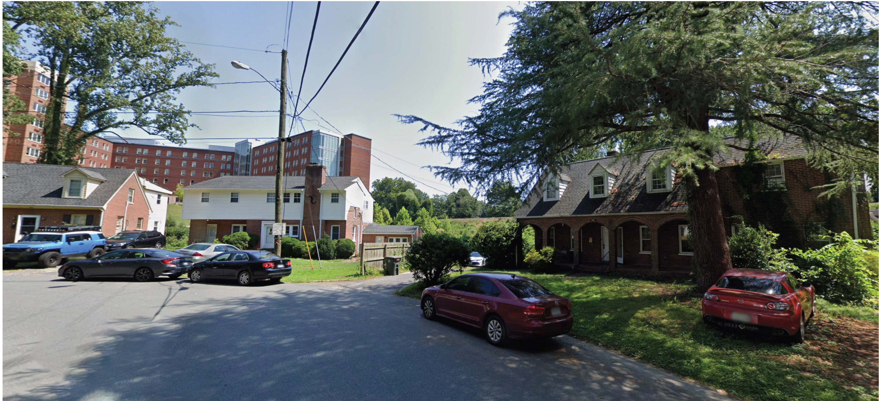
EXISTING VIEW EAST
